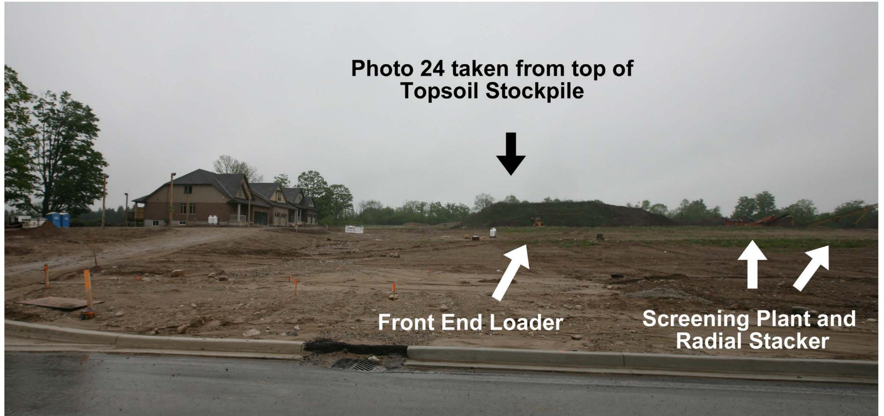
Photo 24a- Photo of stockpile where Photo 24 was taken. Screening plant and stacking conveyor similar to quarry equipment.
